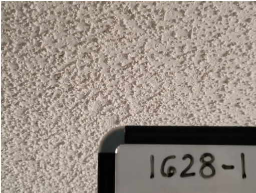
1628-1 Popcorn Texture Typical Interior Ceilings
