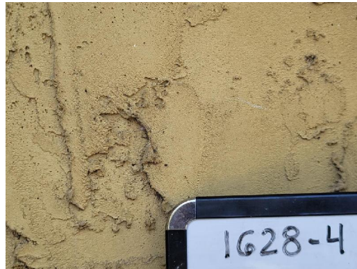
1628-4 Stucco Typical Exterior Walls
