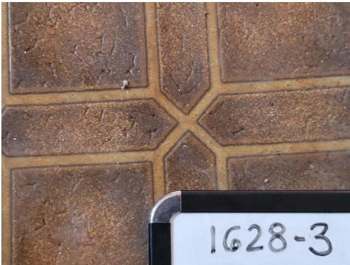
1628-3 Rolled Flooring/Mastic Interior Utility Room
