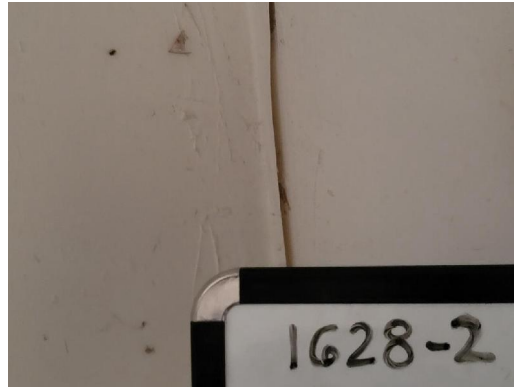
1628-2 Joint Compound/Drywall Typical Interior Walls/Ceilings
